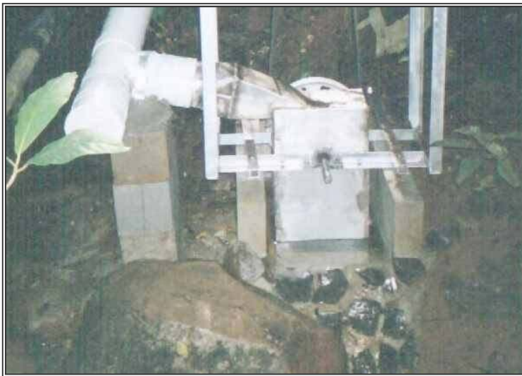
Figure 10 LH6-180 with stainless steel housing & draft tube - note the T-piece arrangement of the penstock adjacent to the turbine to facilitate cleaning
