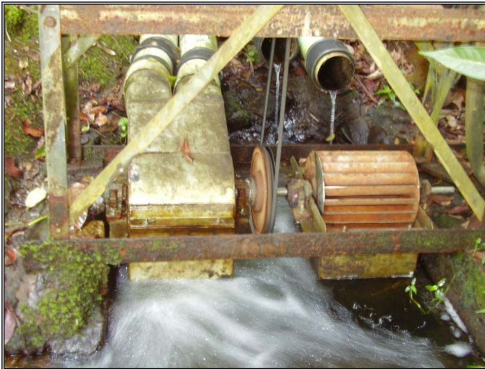
Figure 9 dual LH6-300 Banki-crossflow turbines, end view
